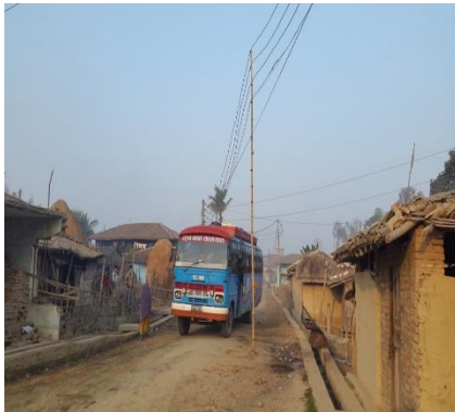
Figure 3: Poorly Managed Wires at Pipariya Kabilasi (The Kathmandu Post, 2019)
